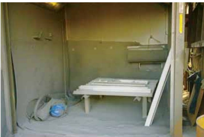
Blasting hood (Sandblasting)
